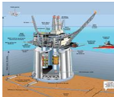
Caisson Retained Island
